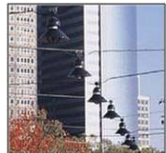
Figure 5.51 Suspended cable lighting.
