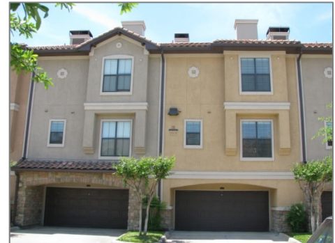
Figure 5.23 Garages integrated into building.
