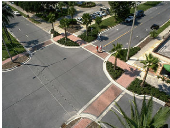
Figure 6.8 Intersection neckdown.
