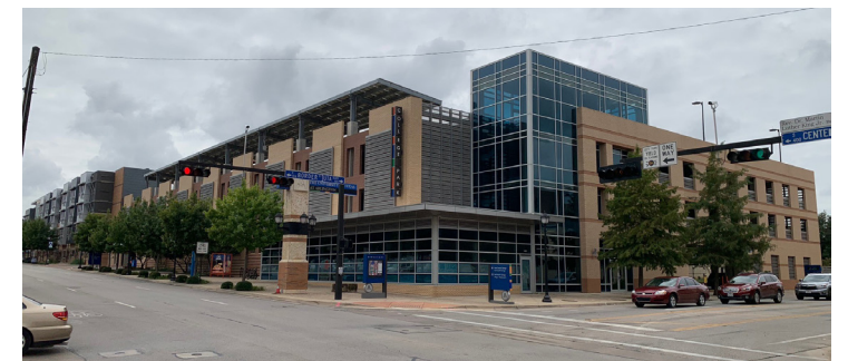
UTA Parking Garage
