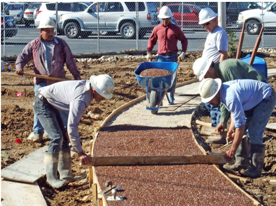
Figure 25: Installation of Filter Pave at the Green at College Park on the UTA Campus
