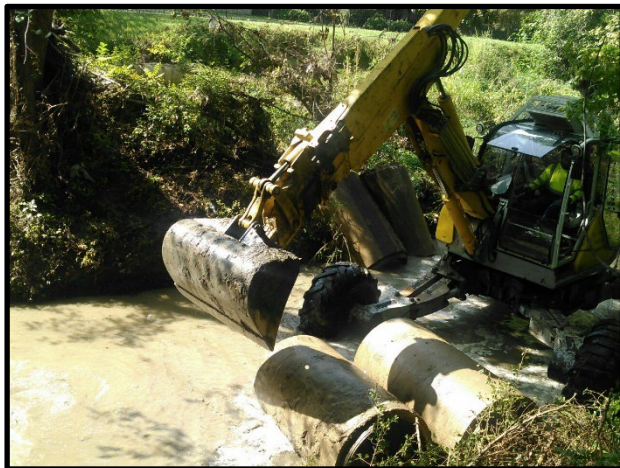
Figure 6 - Removing Broken Storm Drain from a Creek
