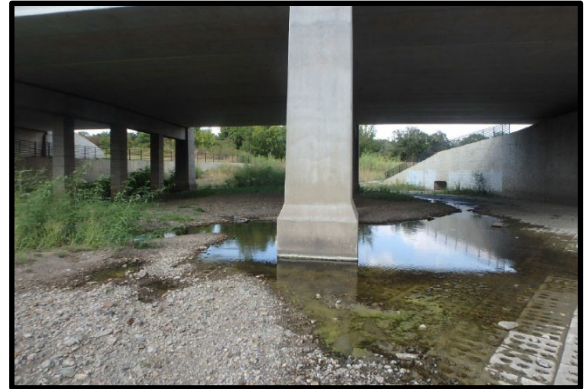
Figure 4 - Photo from Bridge Inspection
