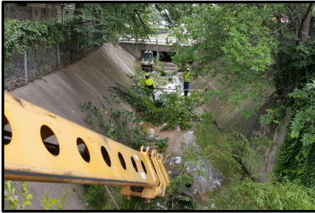
Figure 7 - Vegetation and Debris Removal in Channel
