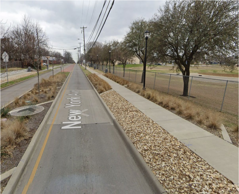
New York Streetscape Improvements from Abram to Arkansas
