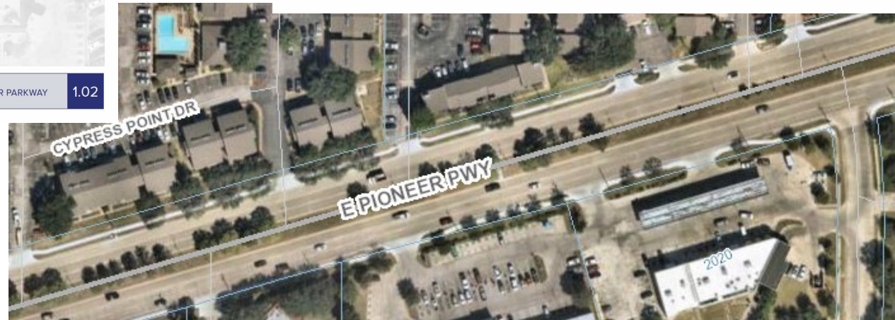
TxDOT Pedestrian Improvements – Completed 2022
