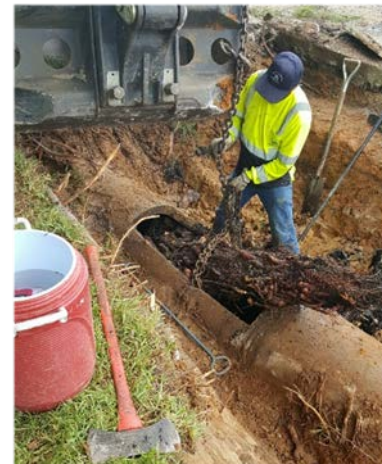
Figure 3.3 Removing a Root Wad From a Storm Drain Pipe
