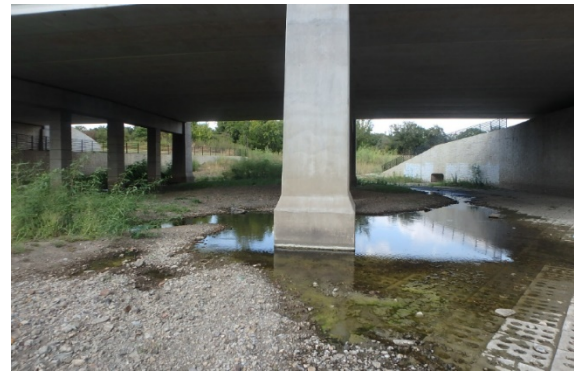
Figure 2.2.2 Photo from Bridge Inspection
