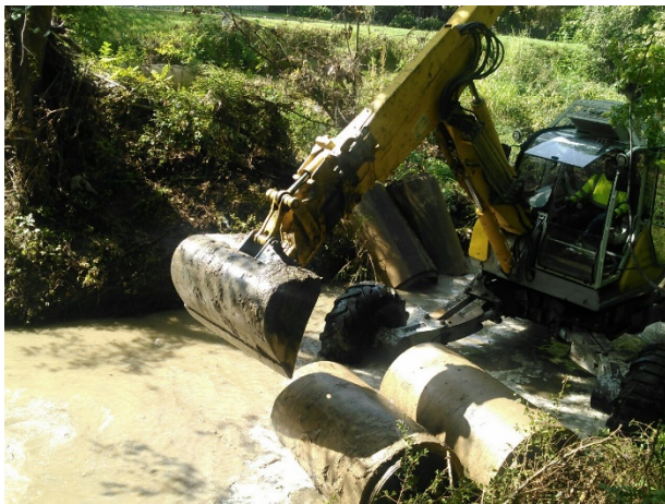
Figure 3.1 Removing a Broken Storm Drain Pipe From a Creek
