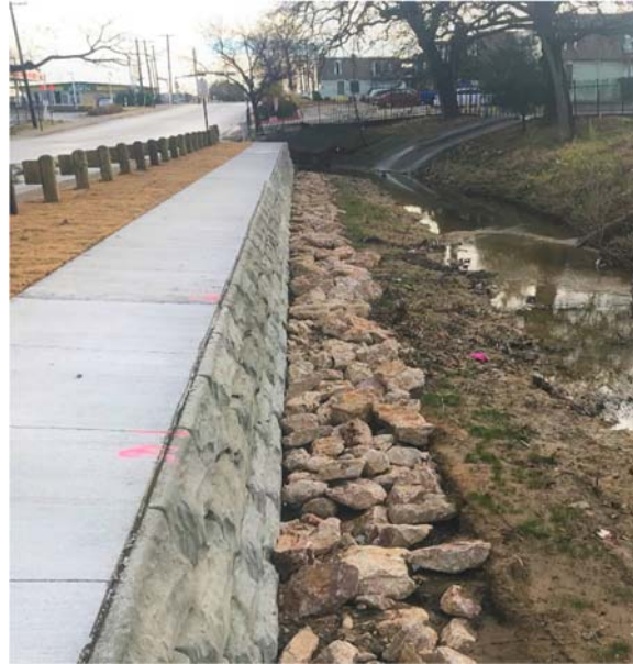
Completed JC-9 Erosion Project
