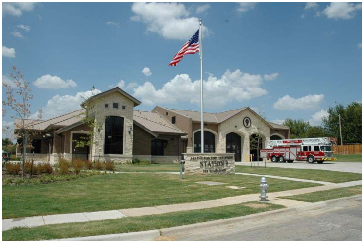
Fire Station 9, which has a LEED Silver designation, was designed in-house by Public Works and Transportation Department staff.
