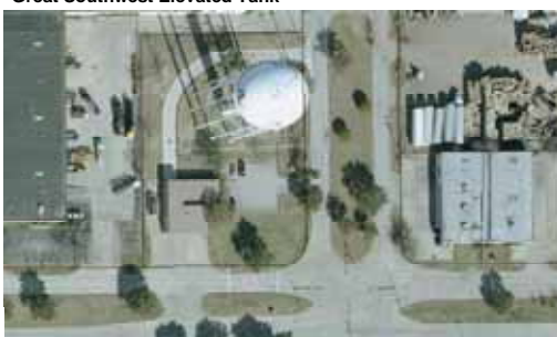
Great Southwest Elevated Tank
