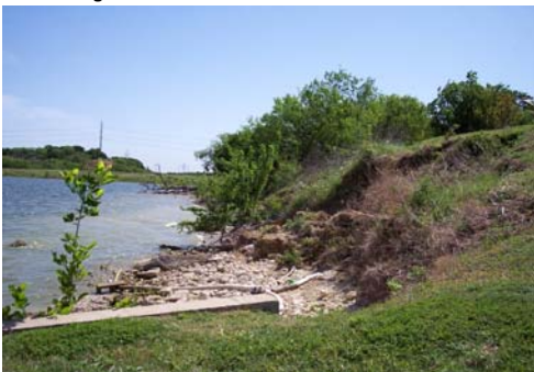
Lake Arlington Bank Stabilization to Protect the Sewer Line
