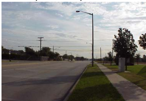
Eastbound Mayfield Road at Sherry Street
