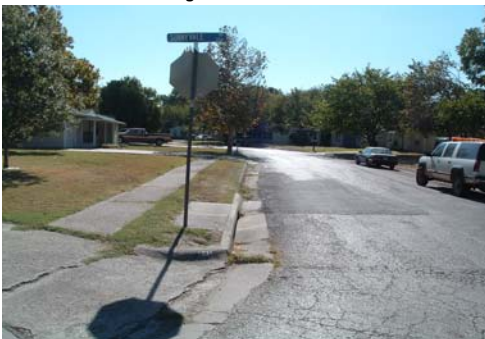
Residential Rebuild Program
