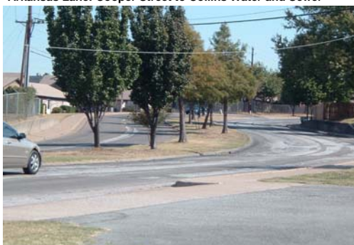
Arkansas Lane: Cooper Street to Collins Water and Sewer
