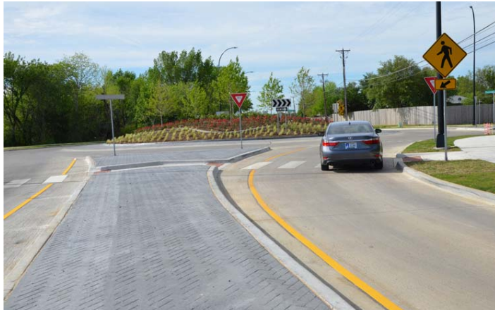
Tri-schools Project Roundabout
